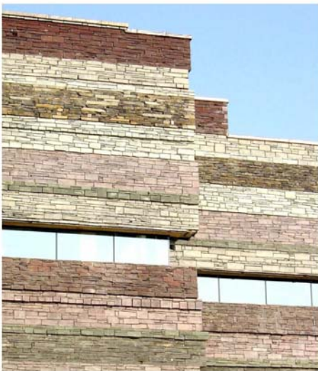
Fig.1 The Staggered Planes of Slate Walling
