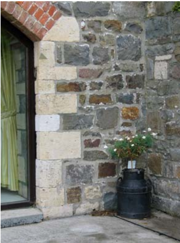
Fig 2. Dundry Stone and Sutton Stone (the white stone 5 th from the bottom) in the former farmhouse opposite the abbey.
